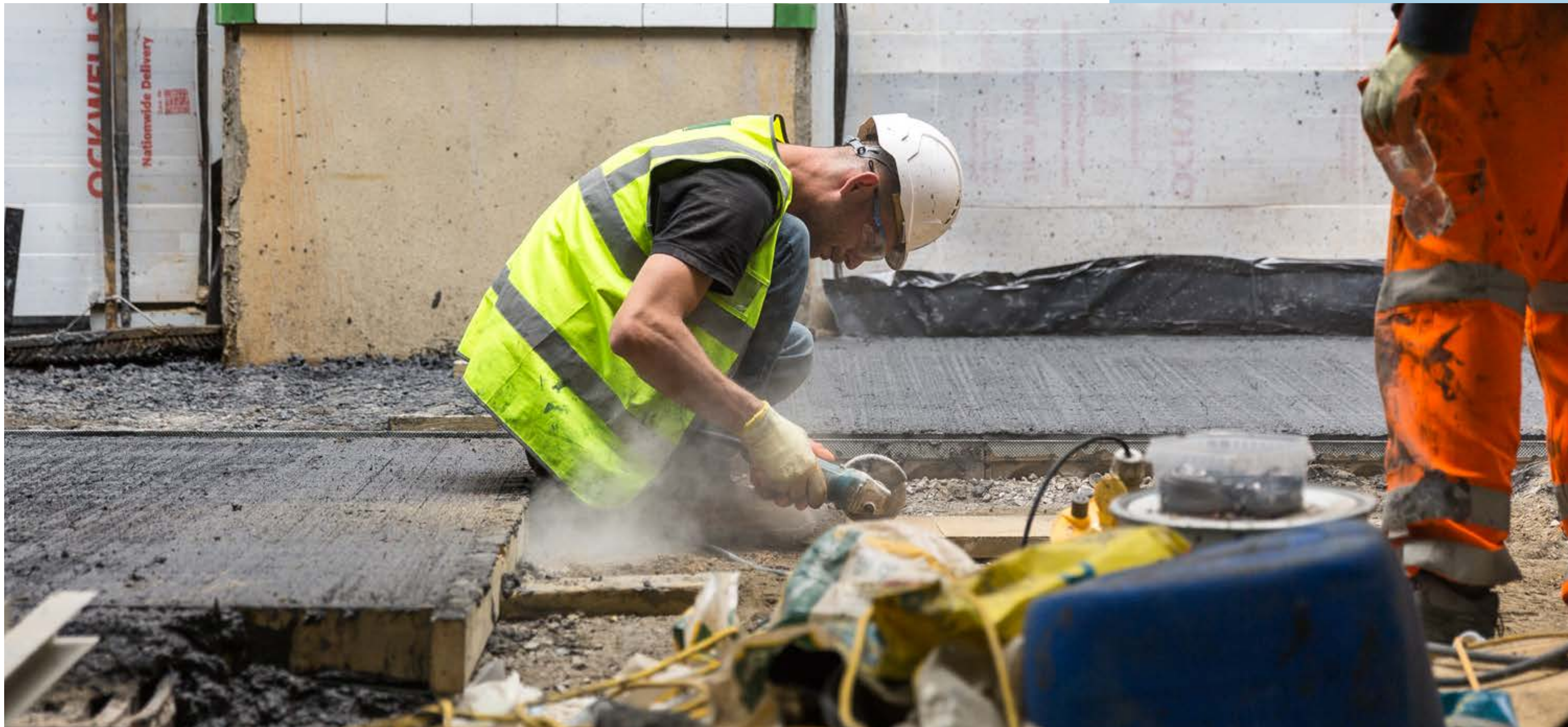
Construction of 27 Eccleston Place, London
